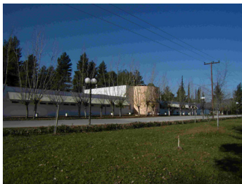
Figure 13: The new spa building (built in the 1960s).
