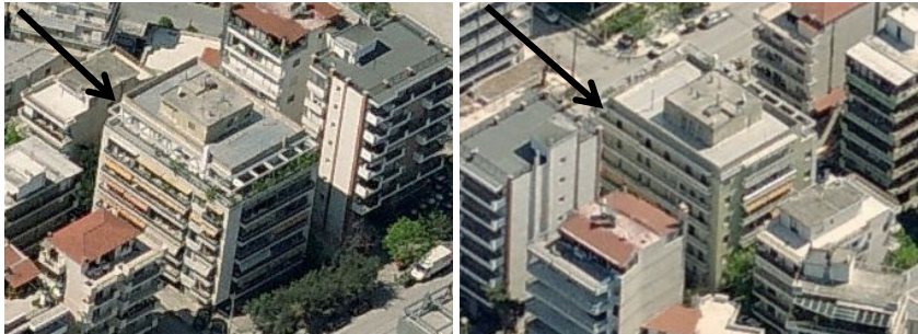
Figure 3: Case study, aerial views of Building B [7]
