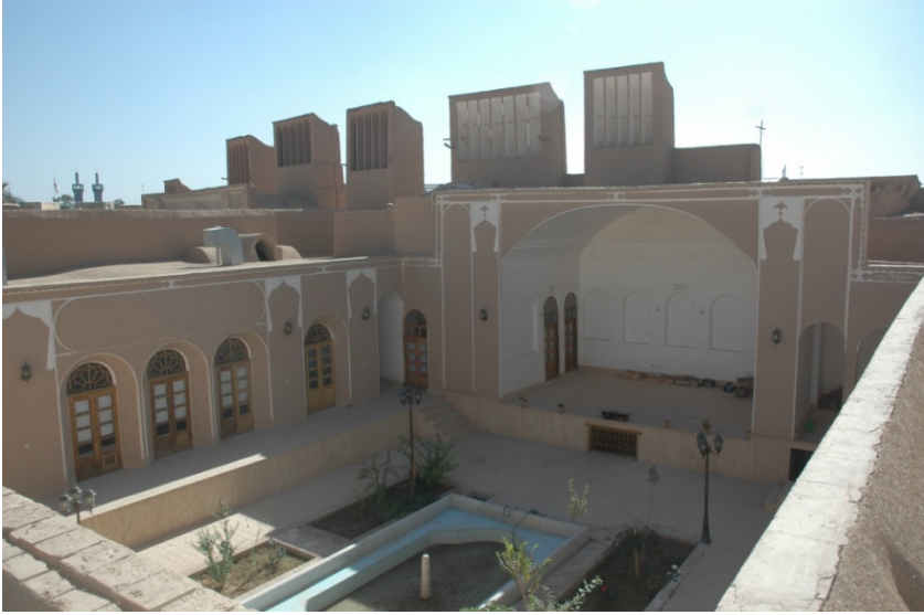
Figure 1: Wind towers, badgirs , as the main cooling system of a house in hot-dry areas by using natural sources of wind, water and vegetation.
