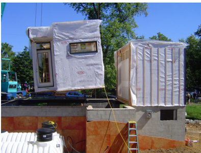
Figure 3: Second of eight modules lowered on basement / foundation.
