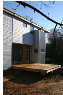
Figure 2: Entry deck of ecoMOD1 house under construction.
