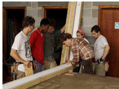
Figure 4: Construction team preparing insulated roof joist.
