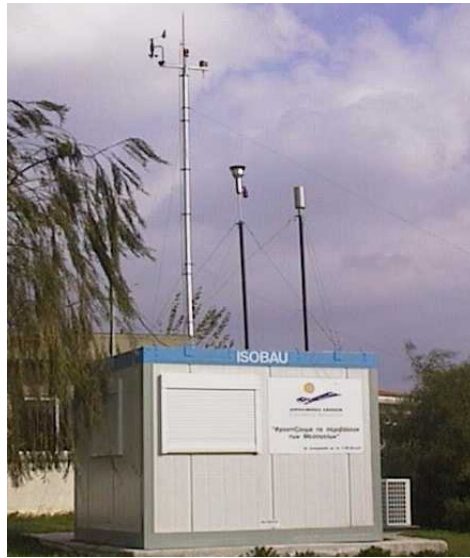
Figure 2: Photograph of the Spata station.
