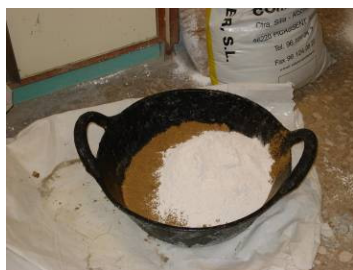
Figure 14: Gypsum mortar preparation.
