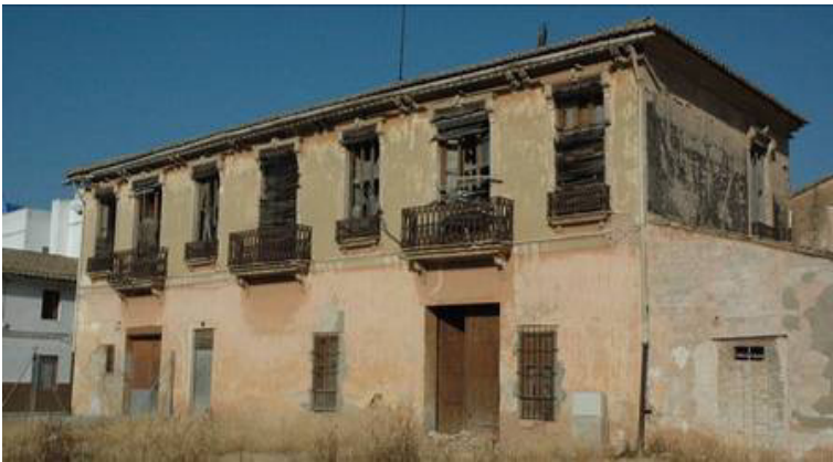
Figure 19: Picanya – historic building. Principal façade (east).
