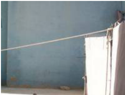
Figure 5: Image of a wall.
