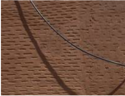
Figure 3: Image of the wall.
