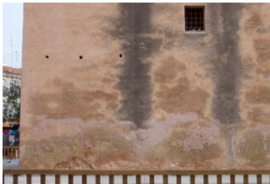
Figure 7: Detail of the tower.
