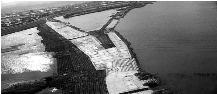
Figure 4.27: The Daijyu dam.
