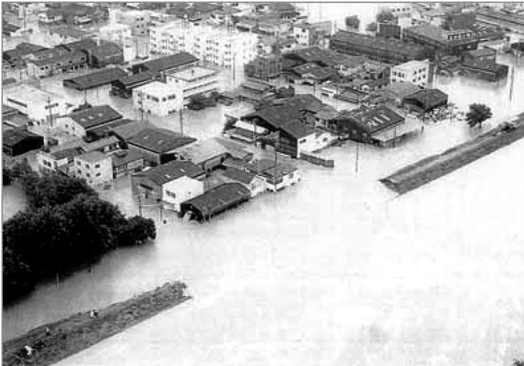
Figure 4.42: The levee break of Shin River.
