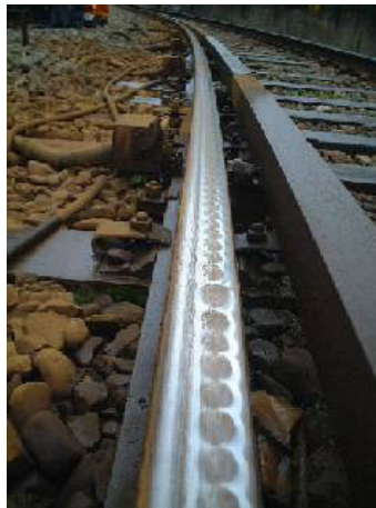
Figure 1: Example of rail corrugation.
