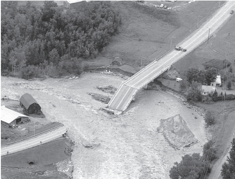
Figure 20: La Baie bridge after the failure of the Ha! Ha! dam.
