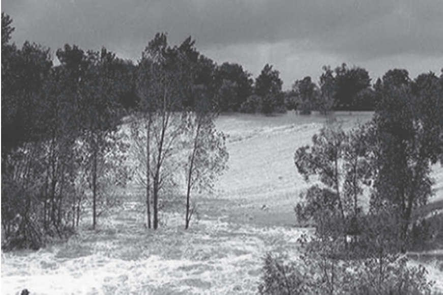
Figure 21: Dam overtopping (available from Association of State Dam Safety Officials website).
