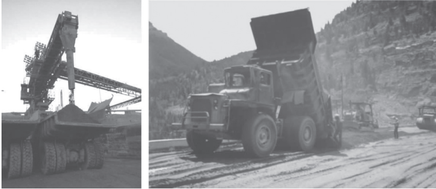
Figure 27: Transportation and placement of RCC.
