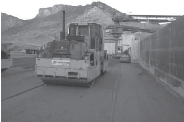
Figure 28: Compaction of RCC.
