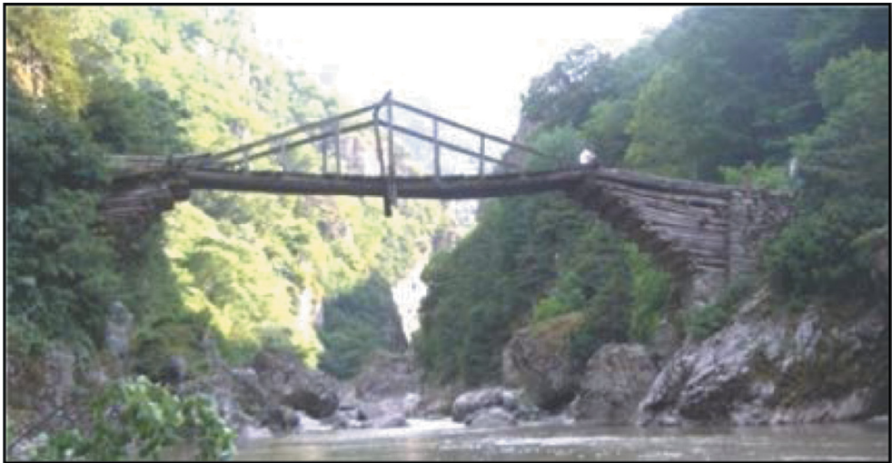
Figure 27: The historical Başkotanı Bridge in Ordu constructed with hybrid system [17].
