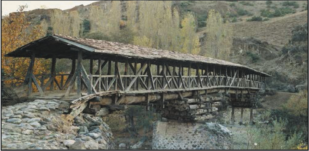
Figure 24: The historical Bayramören Bridge in Çankırı (before restoration) [16].
