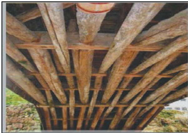
Figure 13: Introdos of main arch of Chinese timber arch bridges (rainbow, woven bridge).
