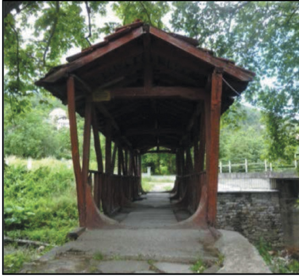
Figure 18: The upper structure of the historical Yakaören Bridge in Kastamonu (Photo credit: S. Yılmaz, June 2016).
