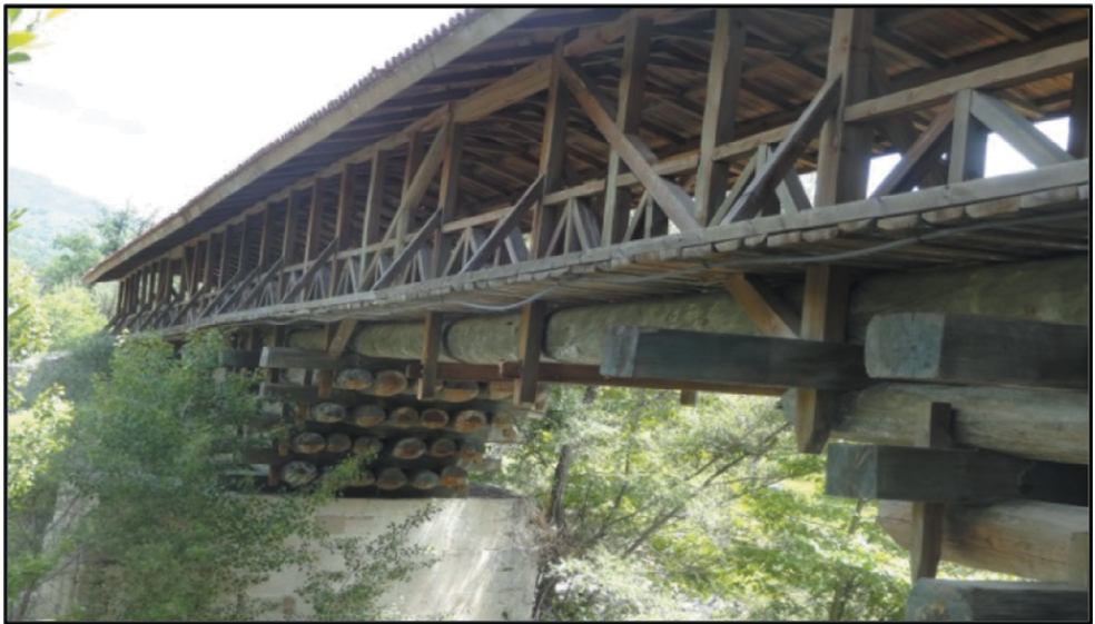
Figure 25: Side view of the historical Bayramören Bridge in Çankırı (after restoration) [16].
