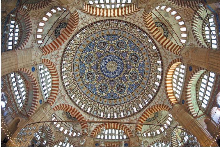
Figure 3: Windows placed around the dome, Selimiye Mosque.
