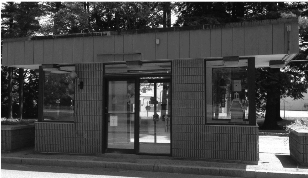
Figure 4: Former guardhouse at Brunswick Naval Air Station. Image by C. Preble.
