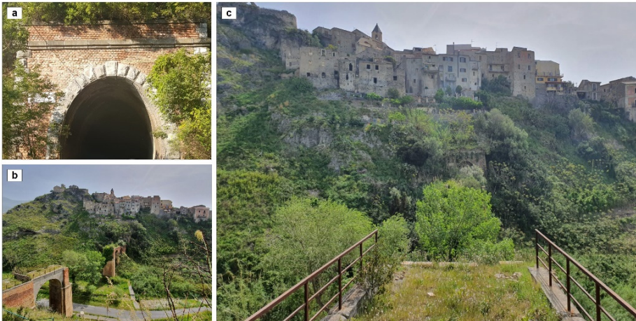
Figure 4: (a) Tunnel close the Cimalonga Tower in Scalea historical center; (b) and (c) Existing railway bridge in Scalea.
