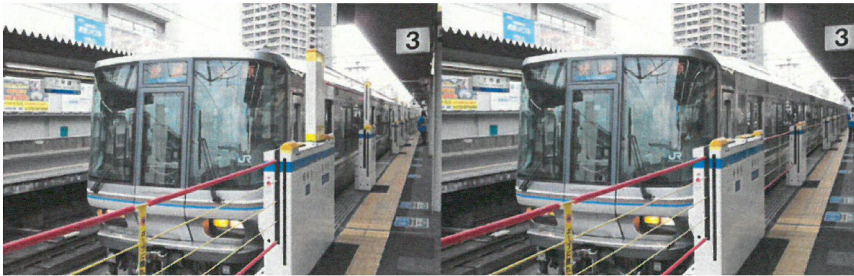
Figure 11: Front view of the wire style platform gates (open/close).
