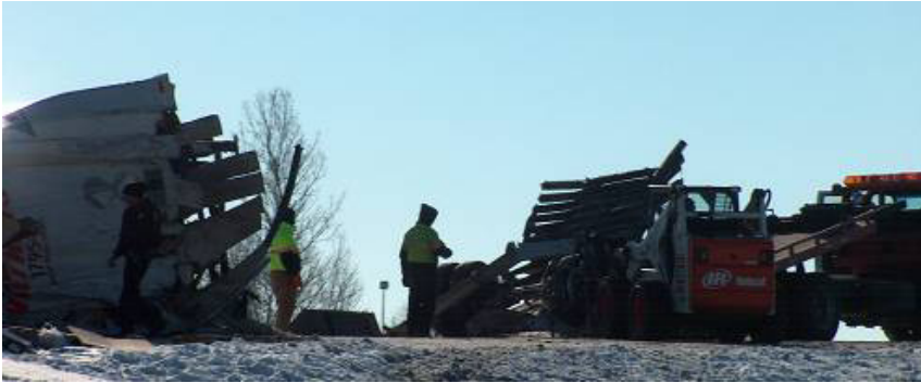
Figure 2: Small back hoe removing spilled cargo from freeway.
