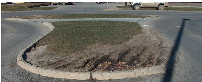
Figure 1: Inadequate-turning radius for trucks.
