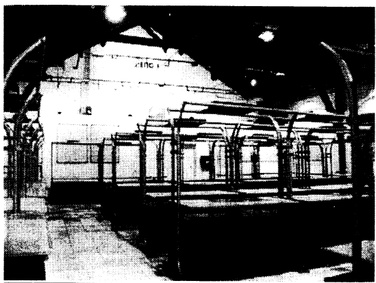
FIG 4: TRAM DEPO, after the reconstruction
