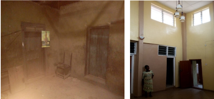
Figure 1: (a) Hall at Lokore house, before renewal; and (b) After renewal; lighting facilitated by clerestory.
