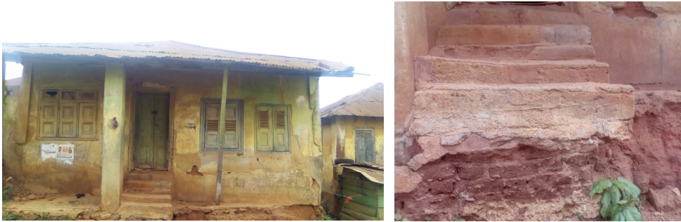
Figure 4: (a) Frontage of Agbedegbede House before renewal; and (b) Close-up of eroded plinth and steps leading into the building, 2020.
