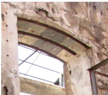
Figure 5: Configuration of a lintel supported by steel beams and concrete plates.
