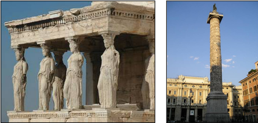
Figure 3: Carved columns which are structural elements themselves (P1) and a column with own seismic behaviour (R1) (in table 3).
