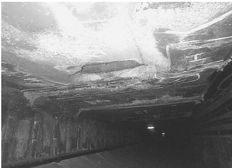
Figure 3: Soffit degradation prior to repair at Queensway Tunnel.
