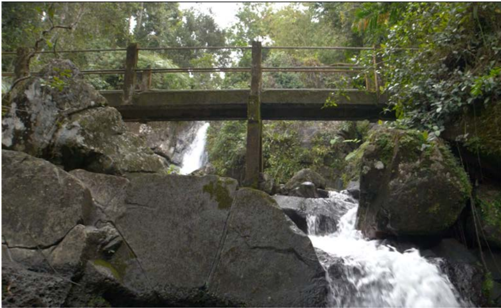
Figure 5: View of La Mina Trail Bridge (looking upstream).
