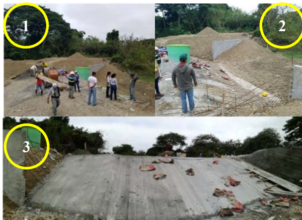
Figure 8: Construction stages of technical-craft dyke.
