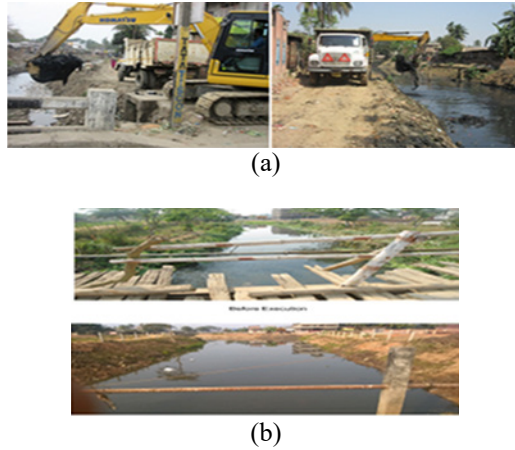
Figure 4: (a) Desiltation of the Mora Bharalu River in progress. (b) Before and after the re-sectioning of the Basistha.
