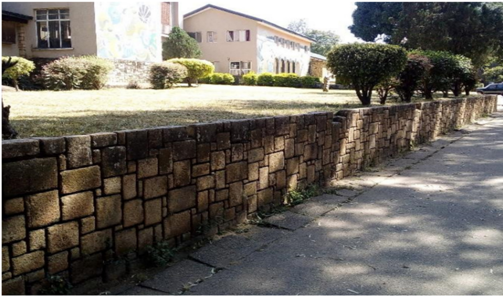
Figure 7: Stones used as retaining wall [23].
