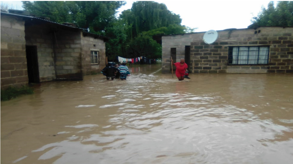
Figure 2: Flooded houses in Maseru in January 2022 [20].
