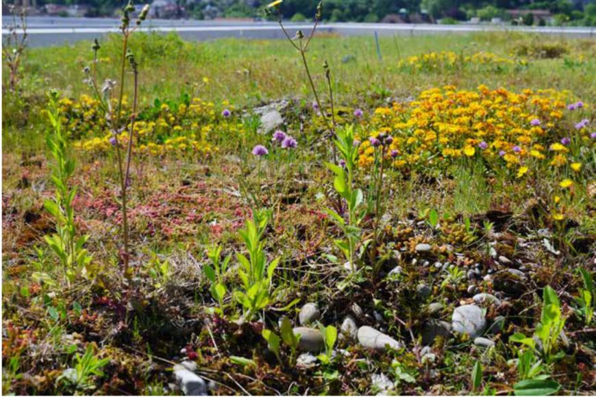
Figure 6: Examples of green roof with herbs, mosses and sedum vegetation. Substrate content and its depth (6–15) are varied over the entire surface of the roof to increase biodiversity (photo: Jonatan Malmberg, Scandinavian Green Roof Institute).
