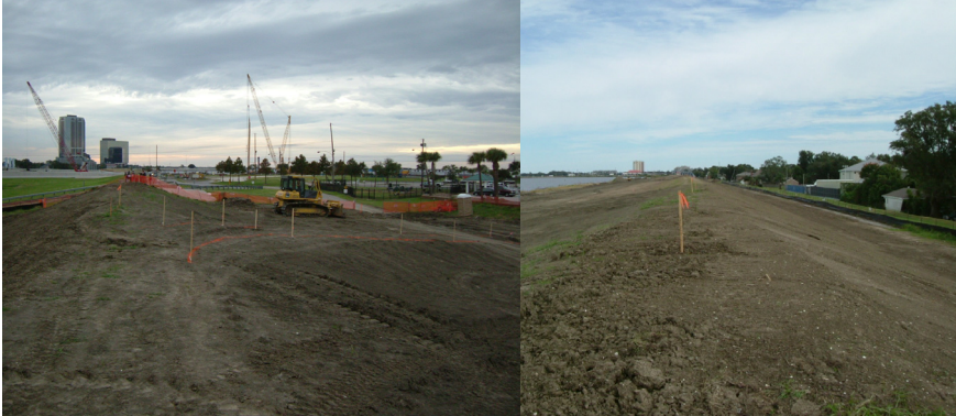
Figure 6: Levee construction and reinforcement.
