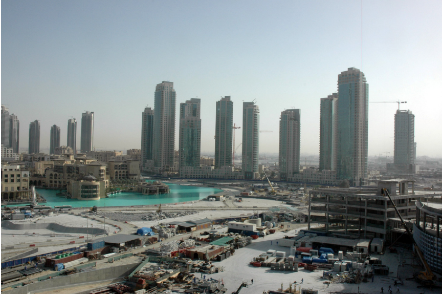
Figure 3: Tall building construction in Dubai (Credit: Paul Armstrong).
