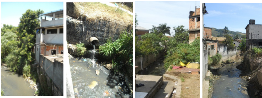
Figure 3: Illegal constructions along Dona Eugênia River (Veról [16]).
