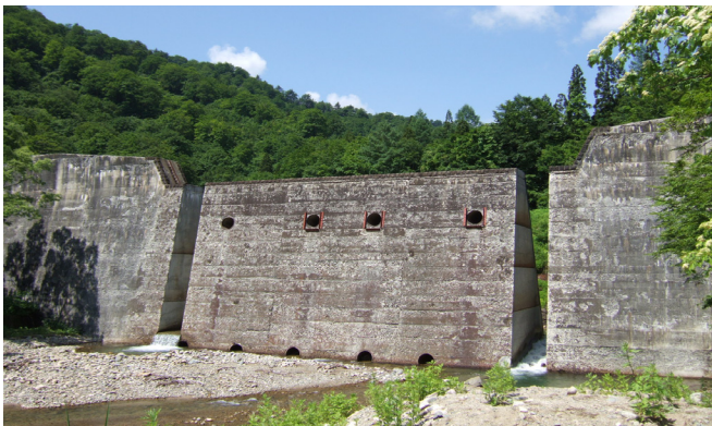
Figure 1: Slit type sabo dam.
