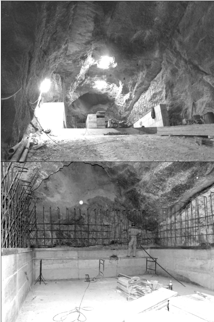
Figure 11: Successive phases of execution of the structures in reinforced concrete.
