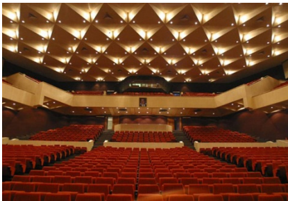
Figure 3: Hall ceiling and the bottom of the split level are totally covered with gypsum board panels.
