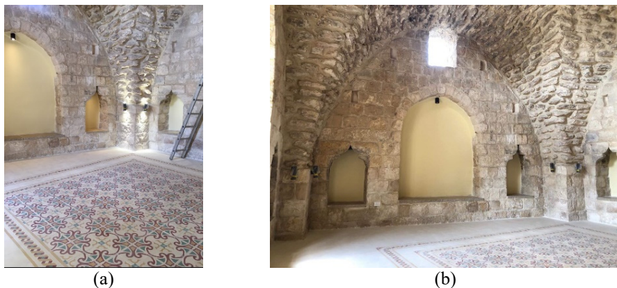
Figure 3: Cross vault in one of the palaces in Anabta, Nablus. (Source: Researcher, 2019.)
