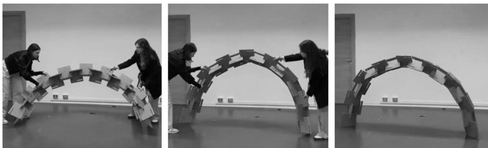
Figure 6: Portion of the archway of the pavilion under construction.
