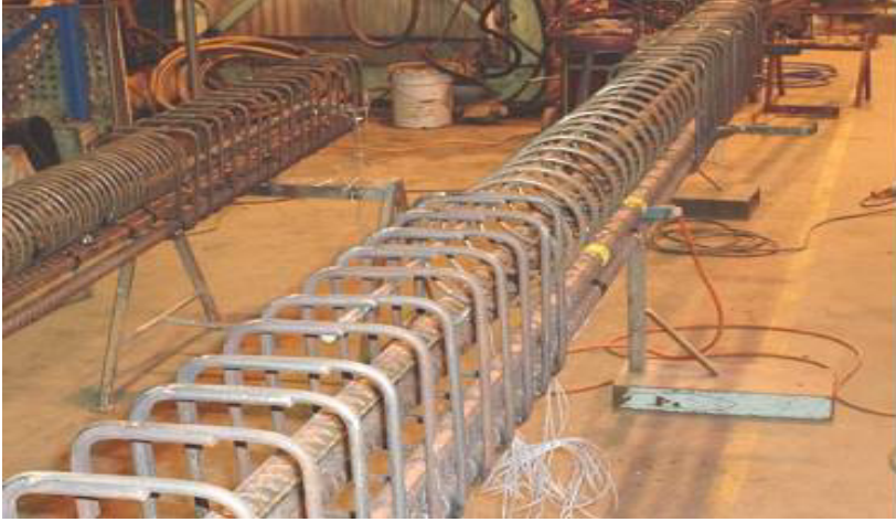
Figure 2: Fixing the helical reinforcement.
