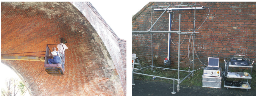
Figure 2: View of the radar measurements. Left: vertical and horizontal profiles under the arch with the 900 MHz antenna. Right: testing area 1 using an automatic 2D radar scanning system with the 1.5 GHz antenna.
