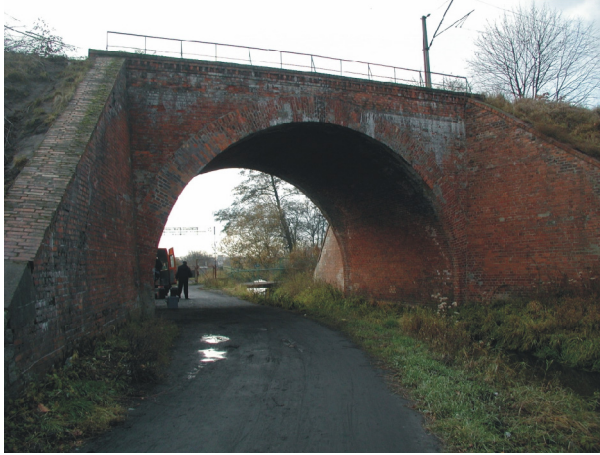
Figure 1: View of the railway bridge from Oleśnica.
