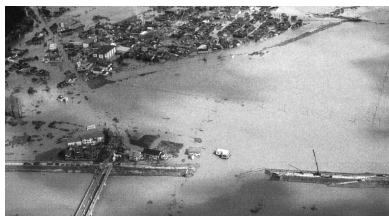
Figure 3: Dike break on the Maruyama River in Toyooka City.
