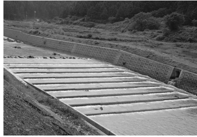
Figure 12: Weir with fish ladder.
