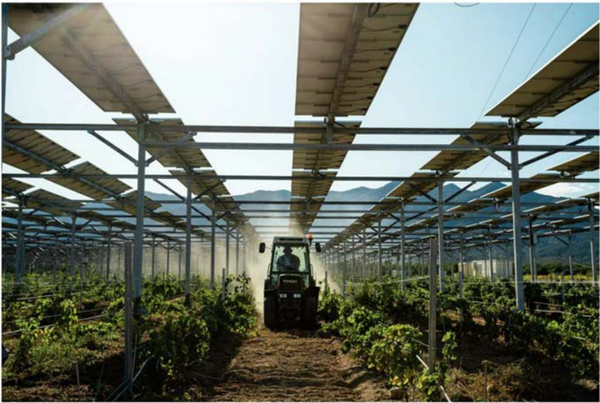
Figure 3: Advanced agrivoltaic installation with raised modules allowing machinery access and crop continuity [15].
