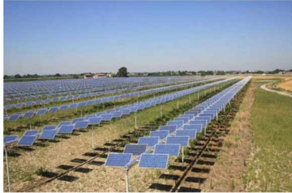
Figure 5: Agrivoltaic plant in Emilia-Romagna with raised modules allowing machinery passage and continuous cultivation [16].
