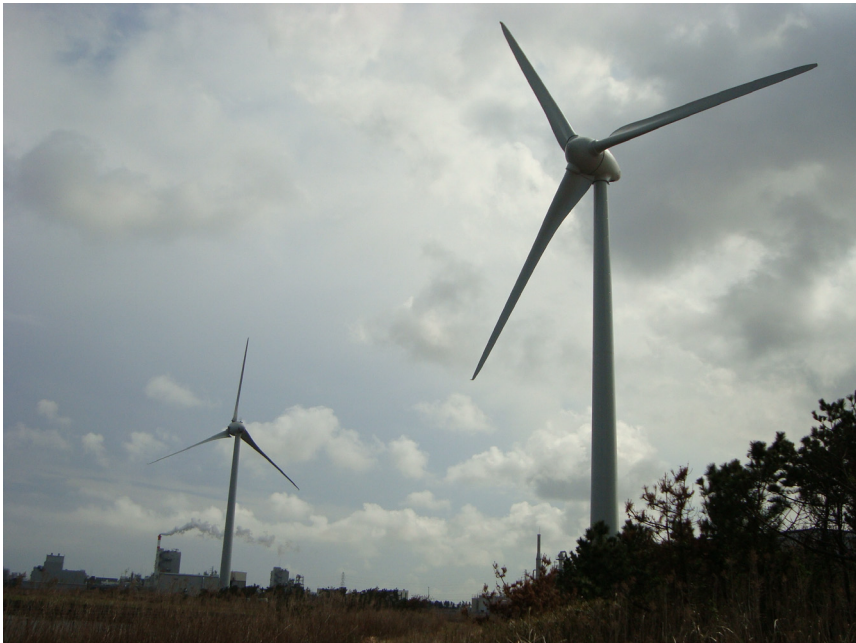
Figure 4: Overview of the wind turbine generator facility (2,300 kW class x 2 sets).
