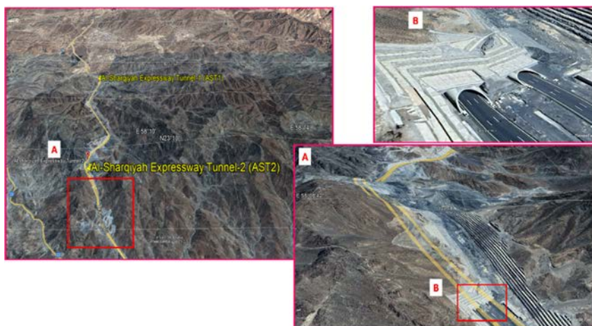
Figure 1: Location of Al-Sharqiyah Expressway Tunnel-2 (AST2), Sultanate of Oman.
