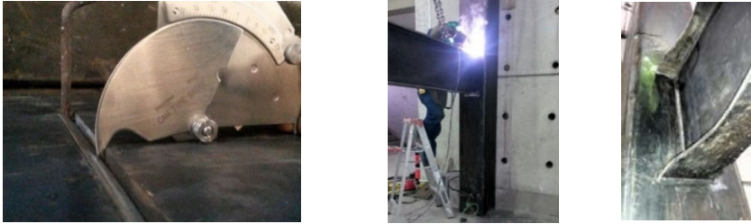
Figure 8: Welding and assembly work.
