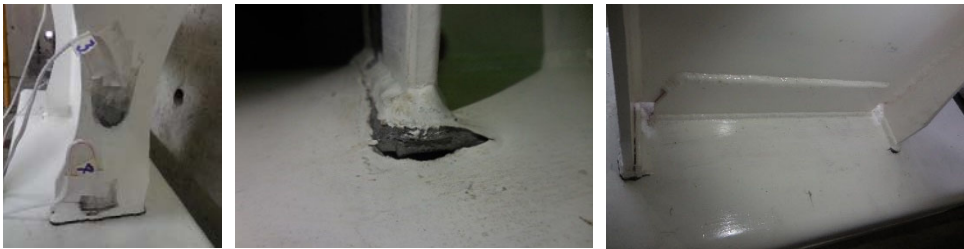
Figure 11: Brittle fracture of continuity plate welds in the experimental test.
