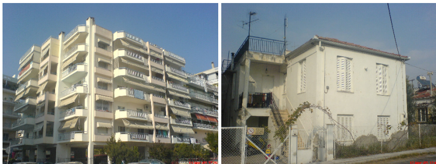
Figure 3: Typical reinforced concrete (left) and masonry (right) buildings.
