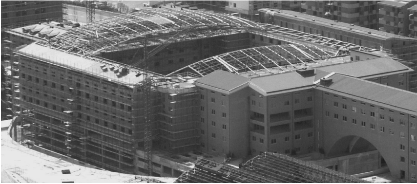
Figure 5: Aerial view of the dome during the launching.
