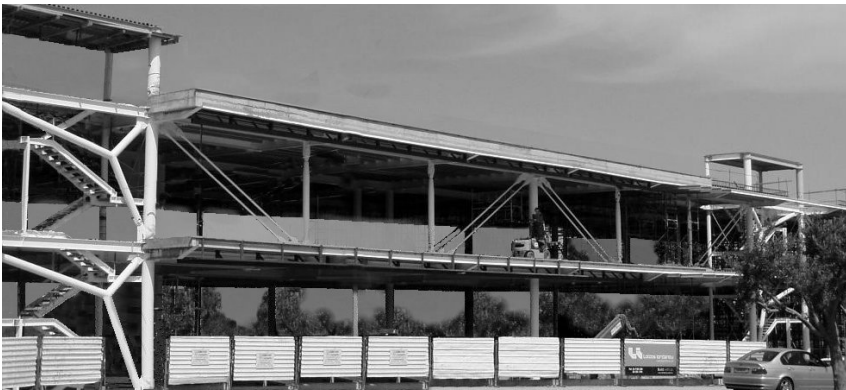
Figure 14: The ITTL longitudinal bracing system.
