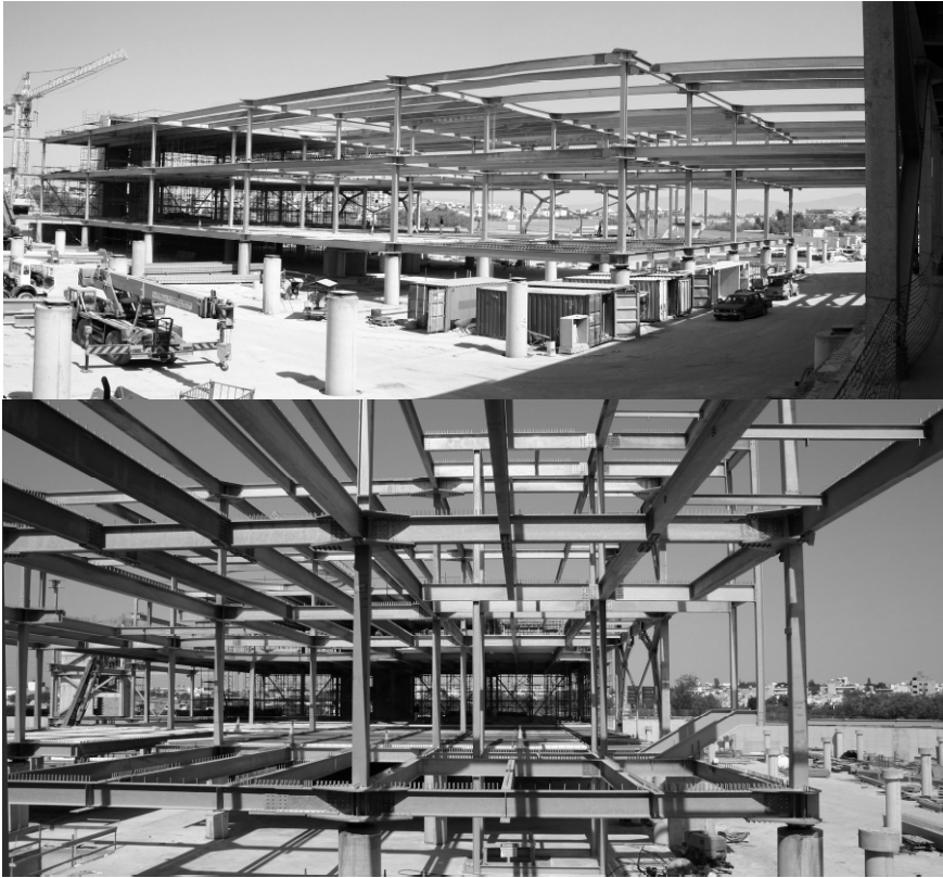
Figure 11: The Shacolas Emporium Park steel skeleton.
