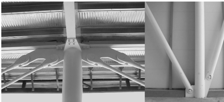
Figure 15: Details of the ITTL 24.00 m span outer girders.
