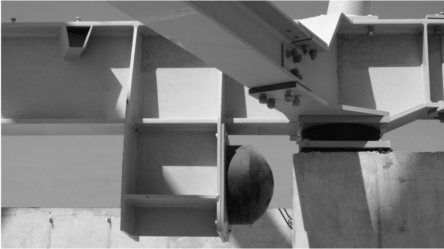
Figure 1: A seismic isolator and the fail-safe system composed of a hemispherical rubber bumper.
