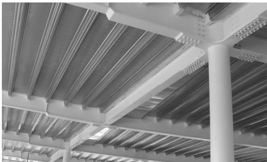
Figure 16: Details of the ITTL 24.00 m span.
