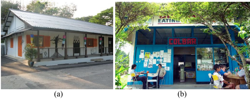
Figure 5: (a) Single storey buildings are created in the new Wessex Village Square. These buildings are designed to look similar to existing ones such as the relocated ColBar (b). (Sources: (a) Fringe Benefit Gallery, http://fringebenefitgallery.com/ , retrieved on 5 Mar 2011 and (b) Colbar, http://epicurative.blogspot.com/2006/04/review-colbar-after-seeing-it-reviewed.html , retrieved on 5 Mar 2012.)
