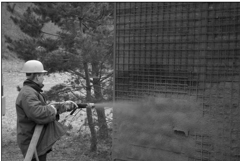
Figure 6: Dust emissions during 3 rd test spraying application.
