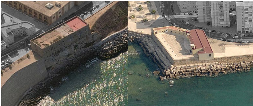
Figure 10: Bastion of San Roque and Bastion of los Mártires.
