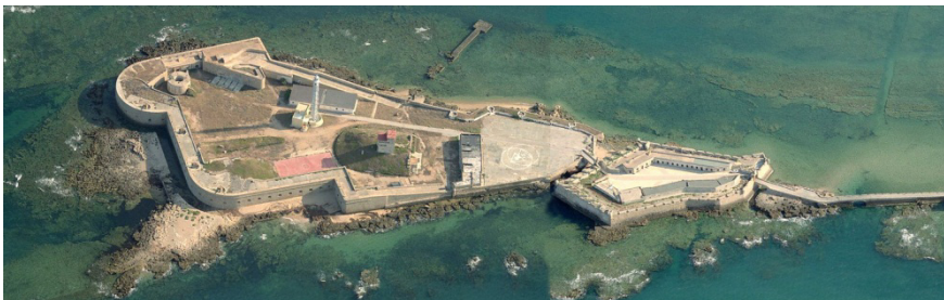
Figure 6: Aerial view of the Castillo de San Sebastián.
