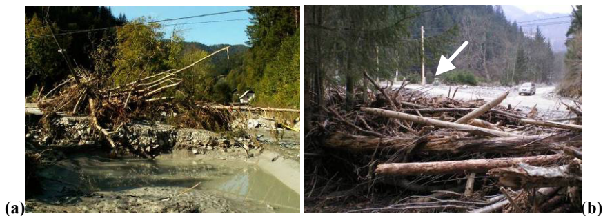
Figure 9: The Davča at the confluence with the Muštrova Grapa: (a) the bridge – not collapsed – from downstream right after the flood; (b) the LW jams trapped at the junction (November 2007). The arrow indicates the bridge location. Source for a: http://www.davca.si .
