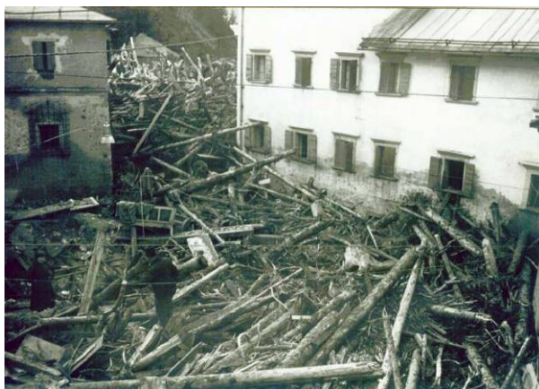
Figure 1: Huge volumes of wood were transported along the Fiorentina river and invaded the small town of Caprile (Italian Alps) during the 1966 flood (R.I. >100 yr).
