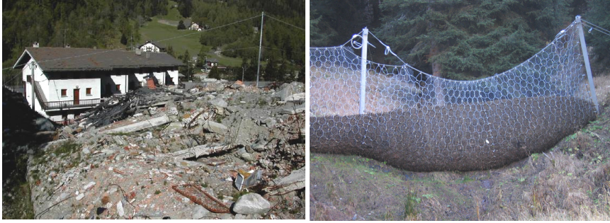
Figure 1: Debris flow deposit directly in front of a building and a filled flexible barrier system.
