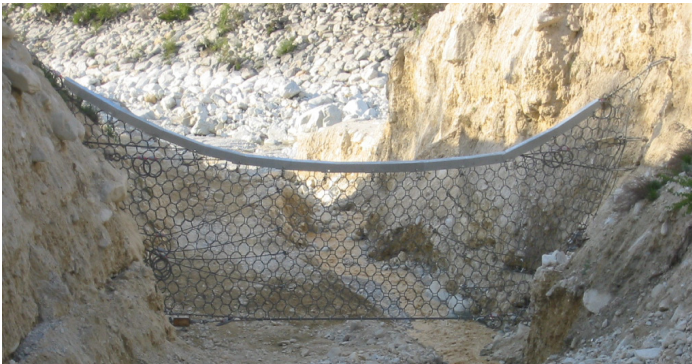
Figure 4: Construction phase and final set up of the barrier 2006.
